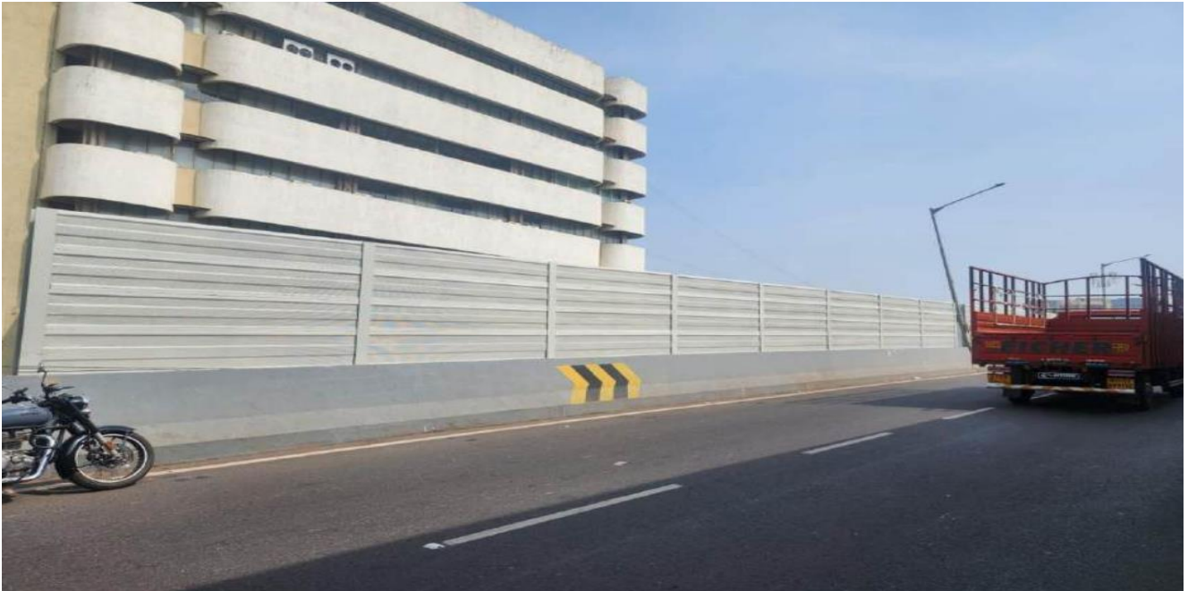
Noise Barriers manufactured and installed at Highway
