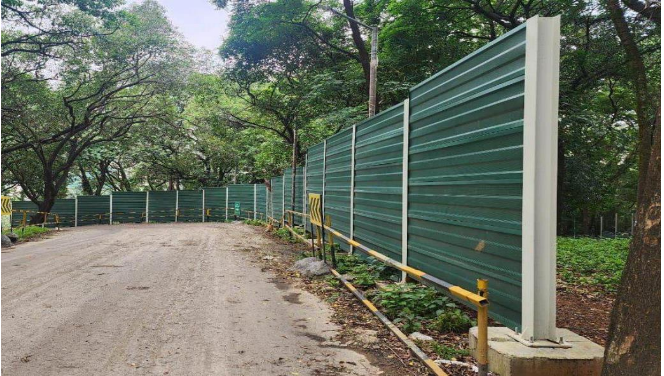
Noise Barriers manufactured and installed at Borivali
