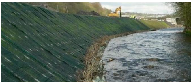
River Bank Protection
