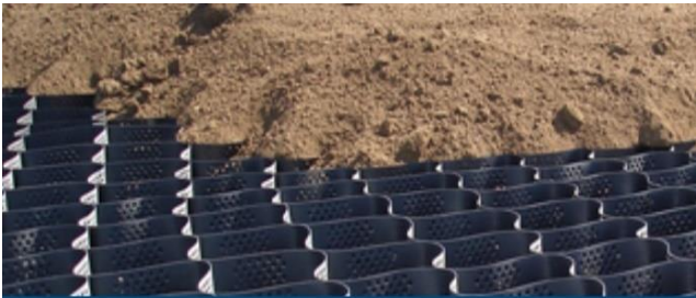
Erosion Control with Geocell
