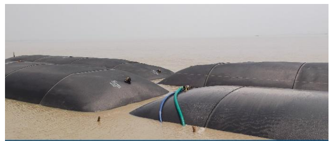
Geotextile Tube for Erosion Control
