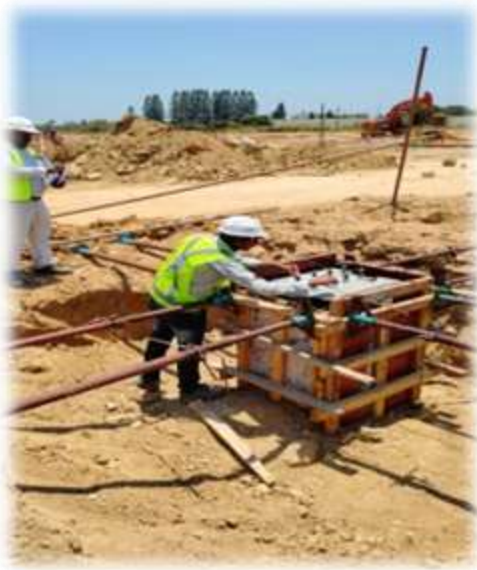
Anchor Bolt Fixing & Checking
