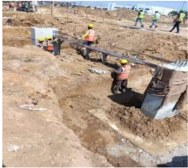
Plinth Beam Shuttering and Concrete Casting
