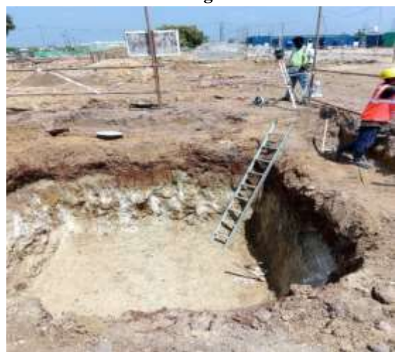
Footing Levelling and PCC Marking Work
