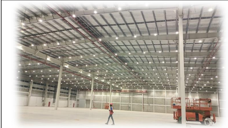
Warehouse - Shakti Infra - Bhiwandi
