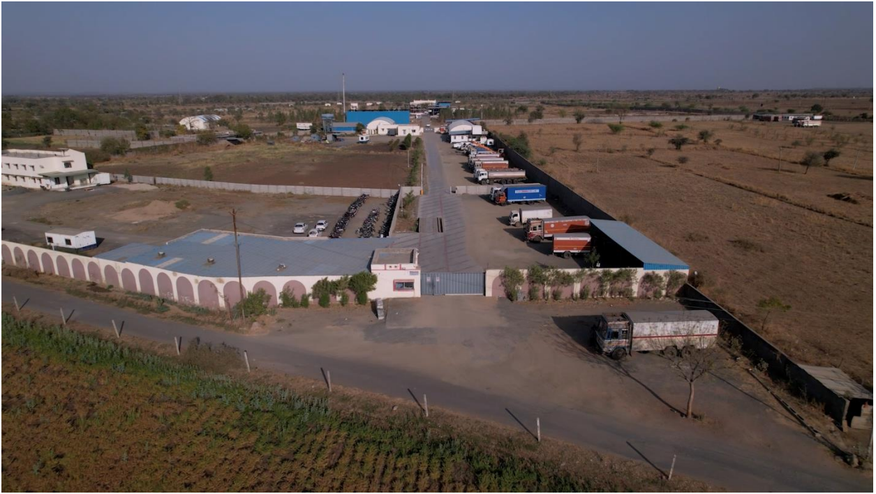
Aerial view of the plant
