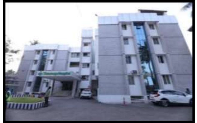
Hospital Main Block
