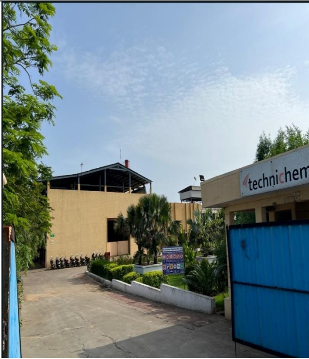
Entrance to Premises
