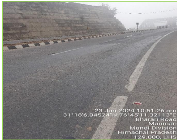
Figure: Rutting
