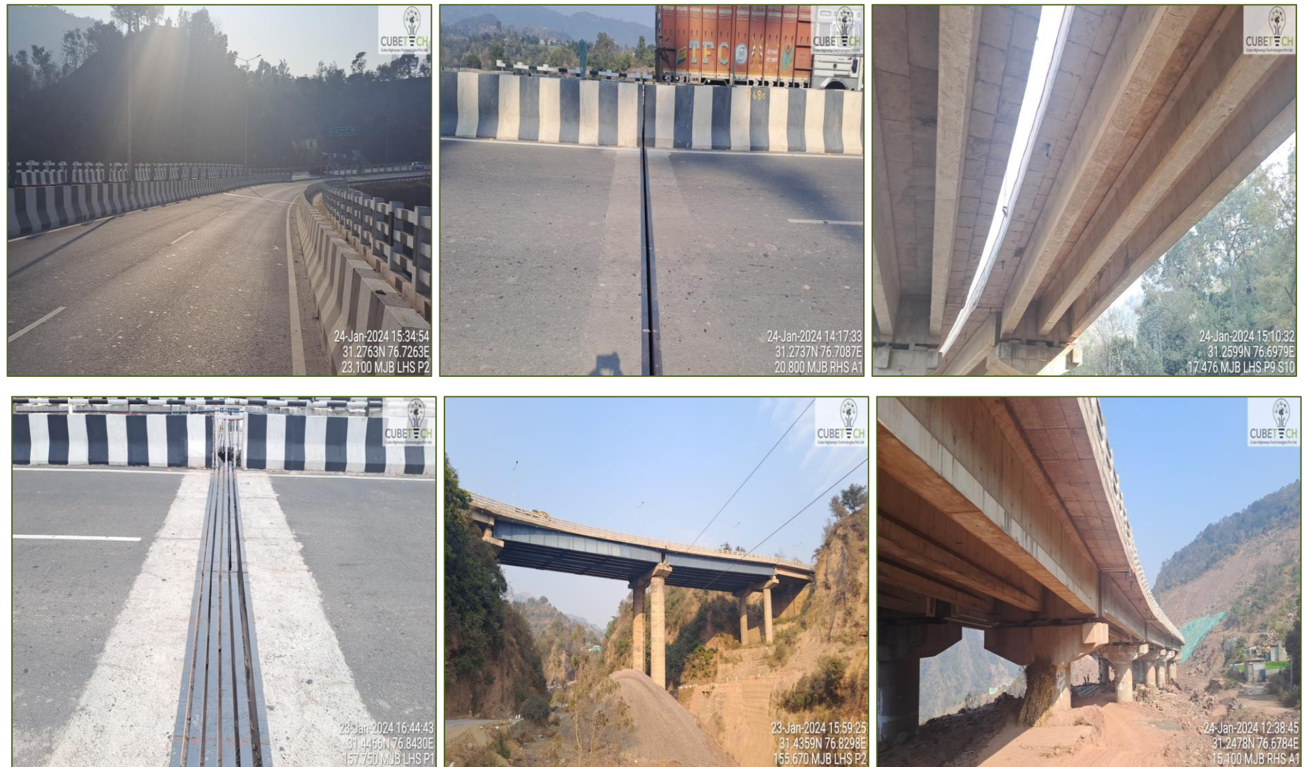
Figure 4-1: Condition of Major Bridge
