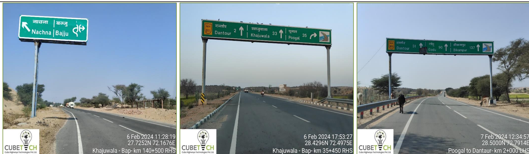
Figure 3-6: Overhead & Cantilever Gantry boards
