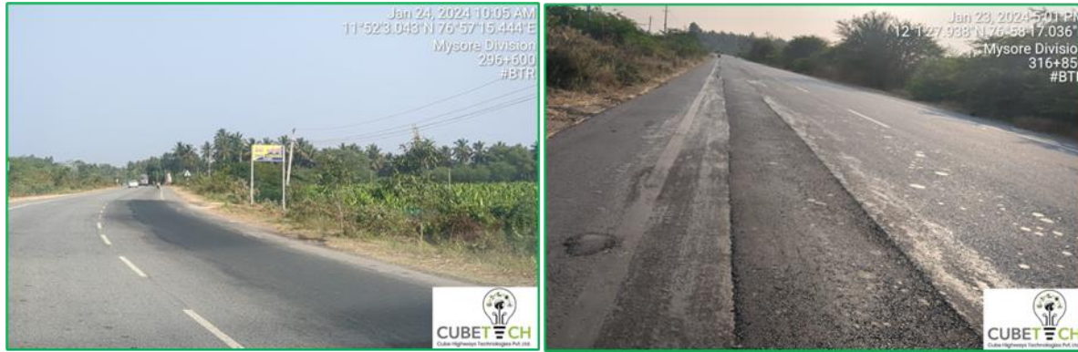
Figure 7-11: Patches
