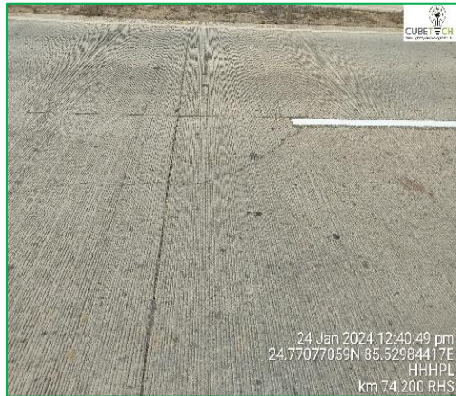
Figure: Corner Break
