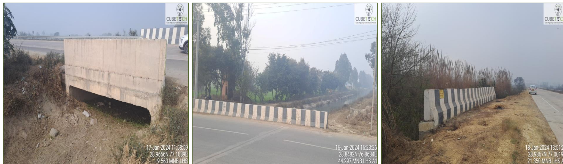
Figure 4-1: Condition of Minor Bridges
