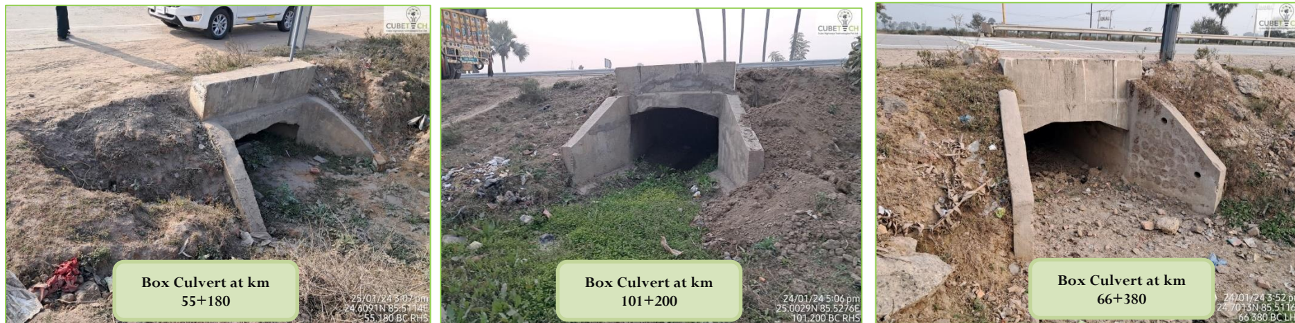
Figure 4-7: Condition of Box Culverts
