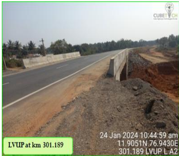
Figure 4-5: Condition of LVUP's
