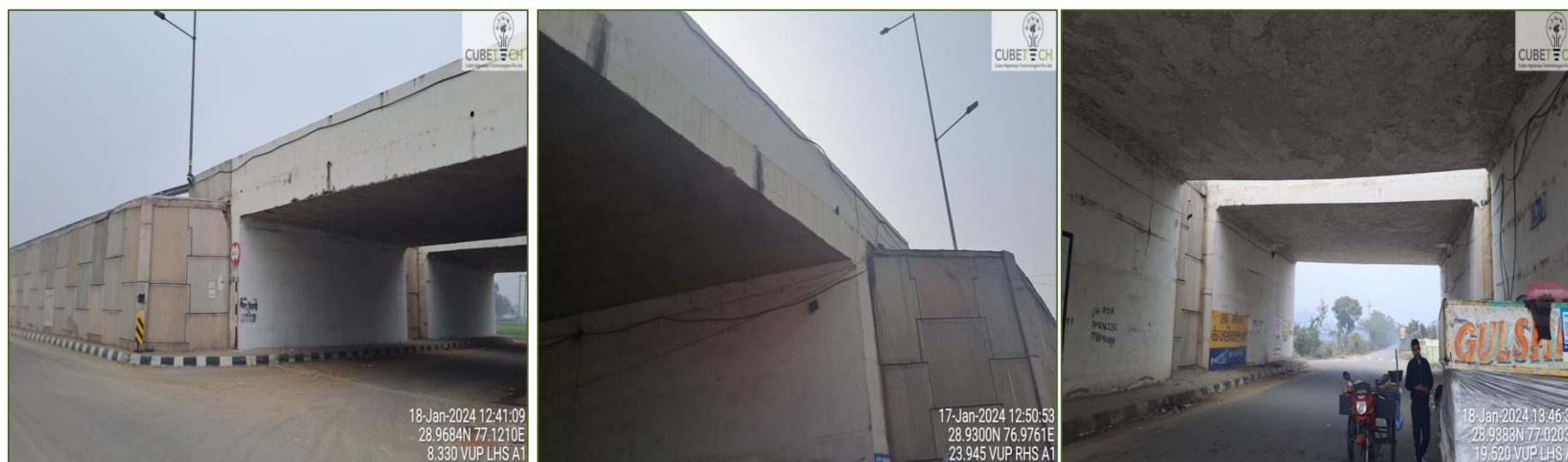
Figure 4-5: Condition of Vehicular Underpasses
