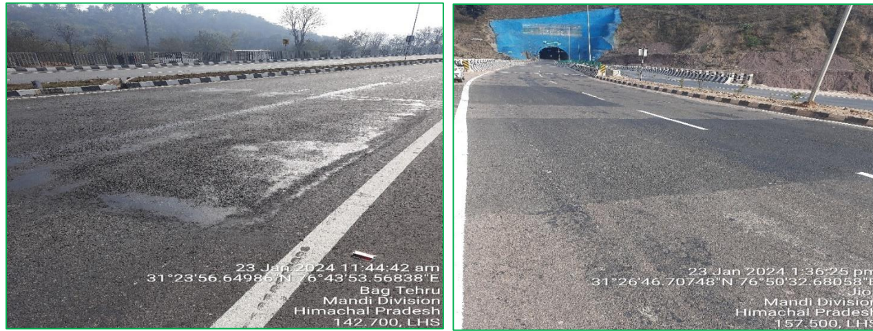
Figure: Patches
