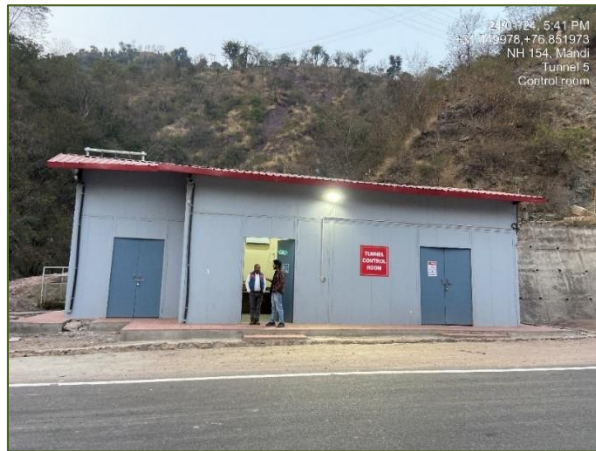
Figure 3-52: Tunnel-5 Control Room.
