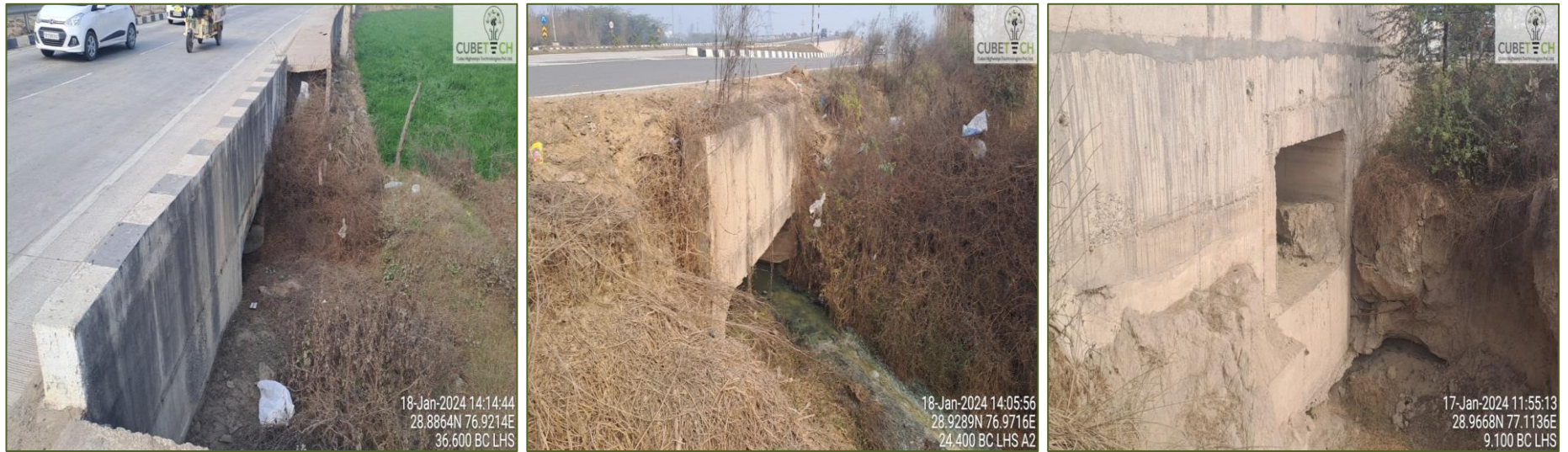
Figure 4-7: Condition of Culverts
