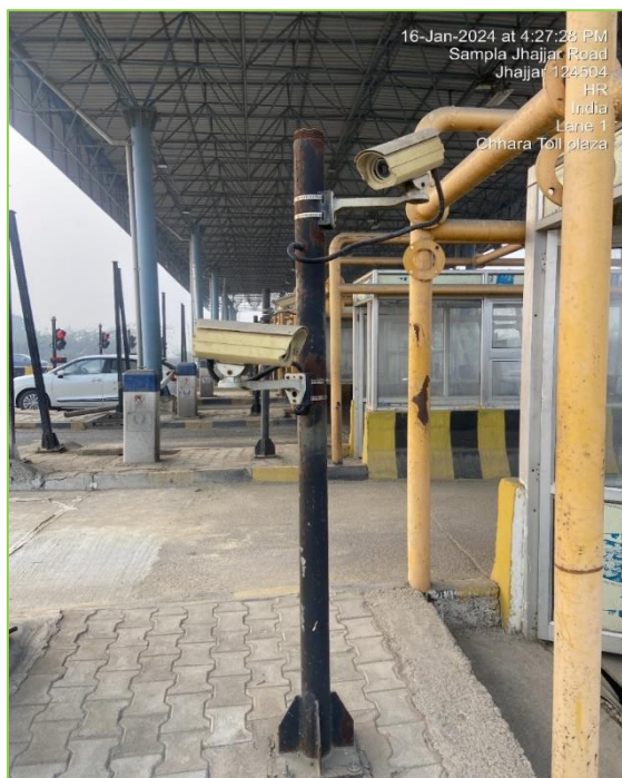
Figure 3-15: LPIC and ICS Cameras.
