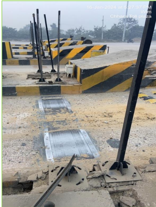
Figure 3-18: Medium Speed Weigh in Motion (MSWIM).
