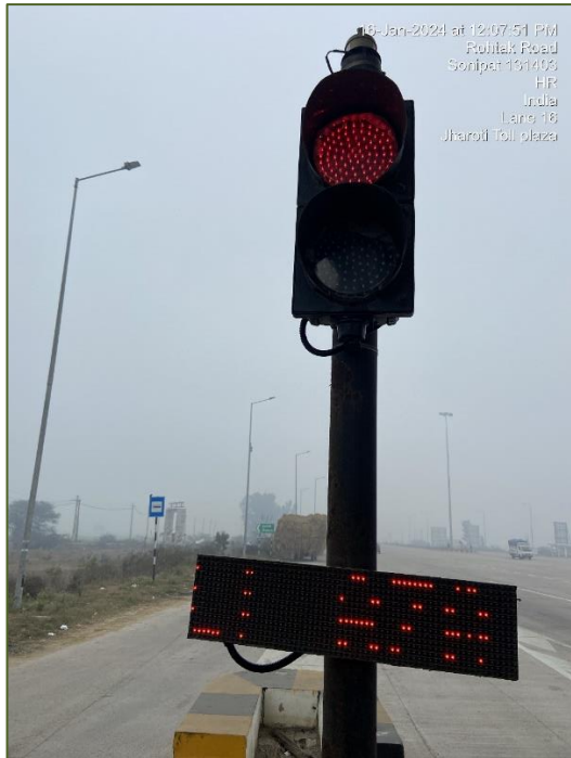
Figure 3-13: Traffic Light (TL) and User Fare Display (UFD).
