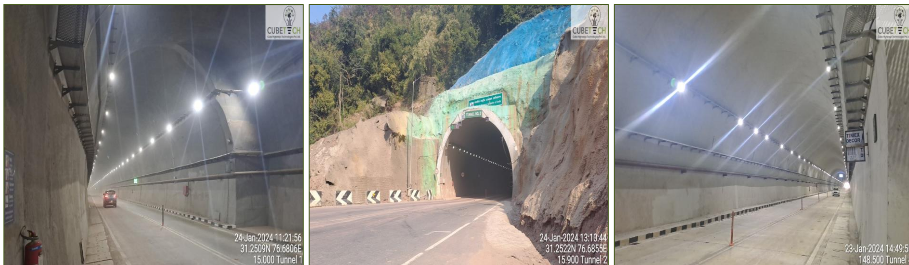
Figure 4-5: Condition of Tunnels
