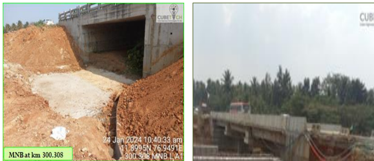
Figure 4-2: Condition of Minor Bridges at km 300+308 & 443+075
