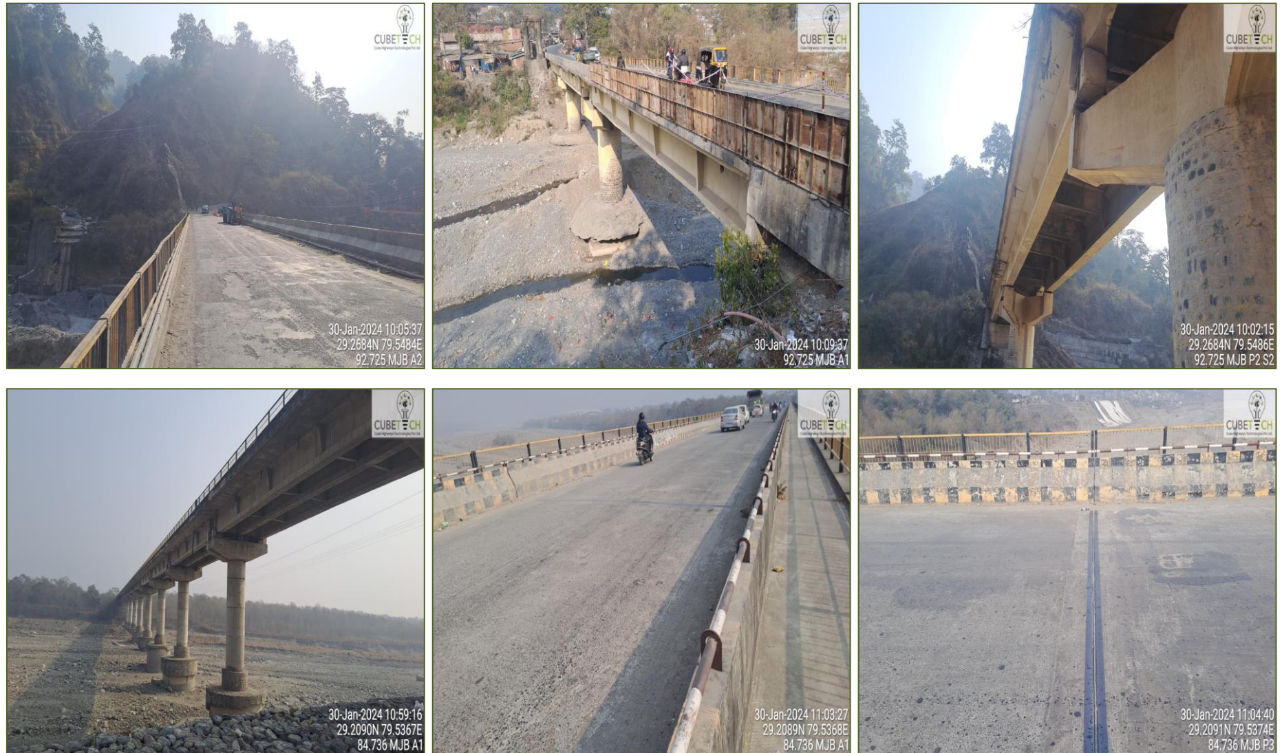
Figure 4-1: Condition of Major Bridges
