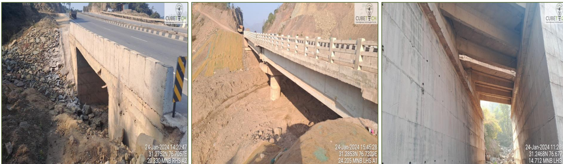
Figure 4-2: Condition of Minor Bridge
