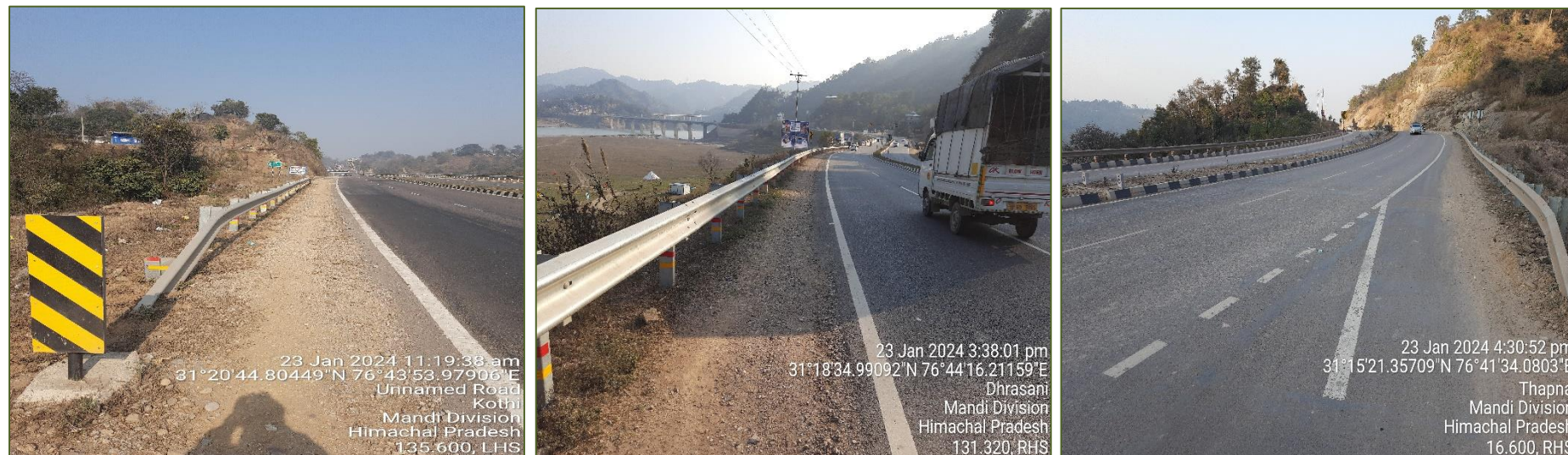
Figure 3-4: Safety crash barrier (MBCB) along the project stretch
