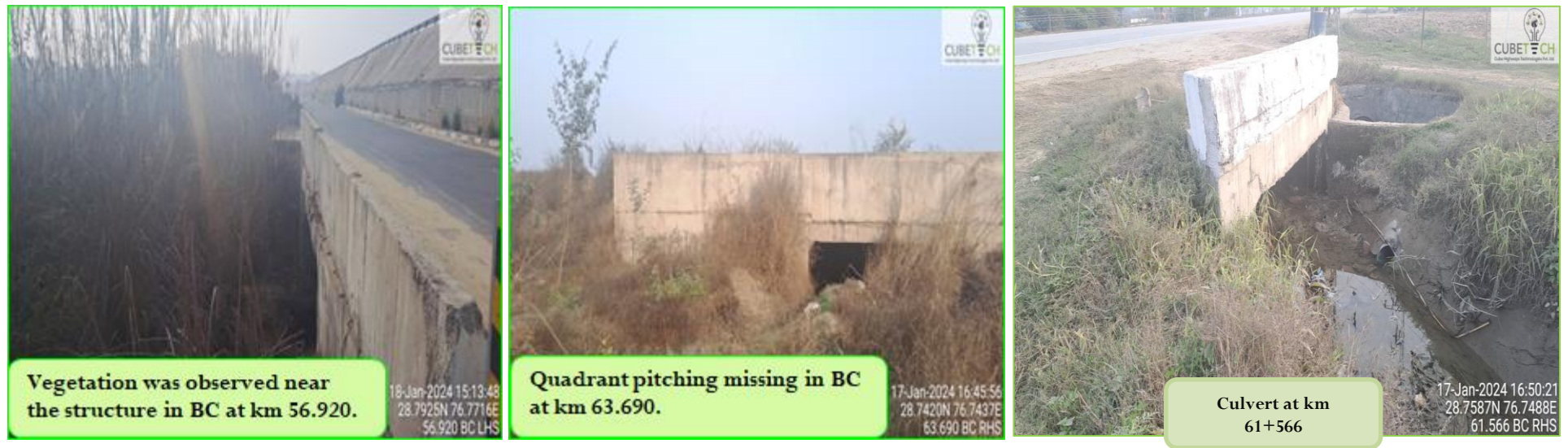
Figure 4-6: Condition of Culverts
