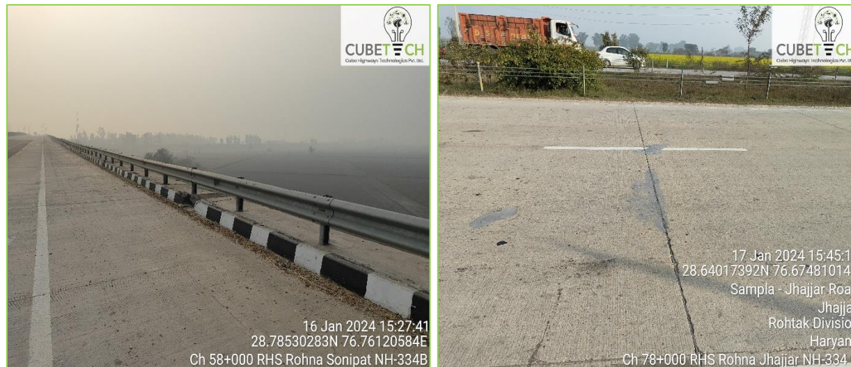
Figure 3-4: Crash barrier along the project stretch
