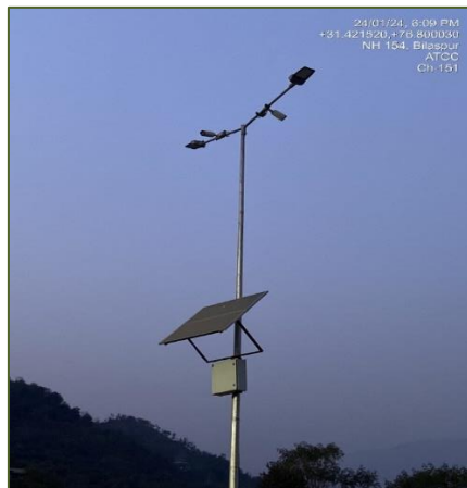
Figure 3-27: Camera Based ATCC.
