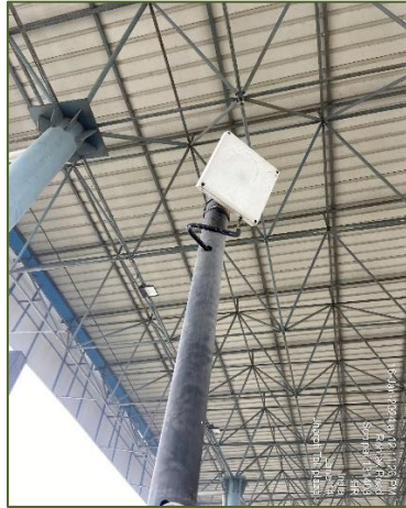
Figure 3-8: RFID reader.
