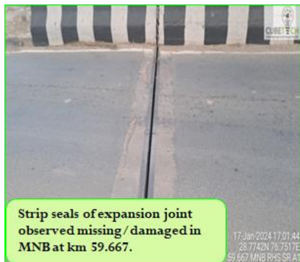
Figure 4-1: Condition of Minor Bridges
