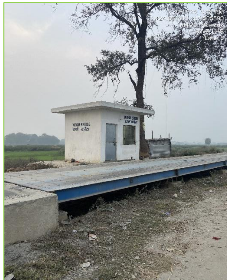
Figure 3-23: Medium Speed Weigh in Motion (MSWIM).
