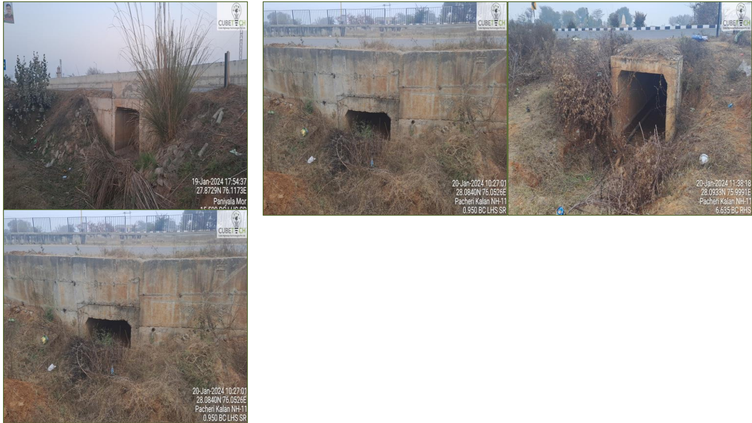
Figure 4-5: Condition of Culvert
