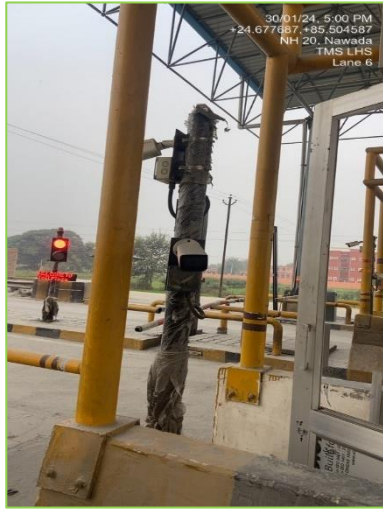
Figure 3-20: LPIC and ICS Cameras.
