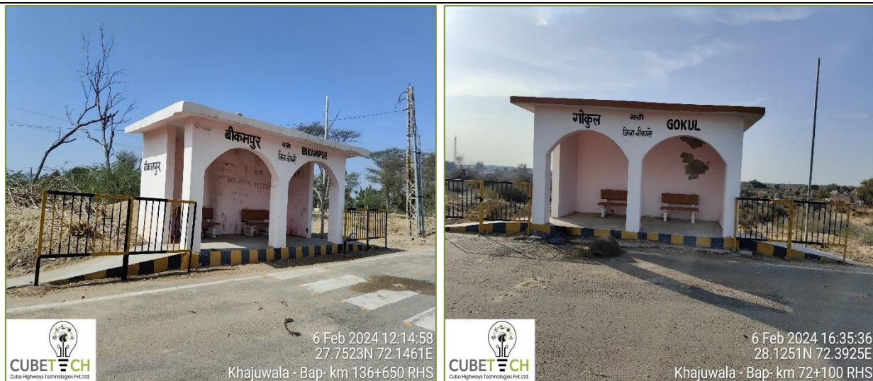
Figure 3-10: Bus bays / shelters
