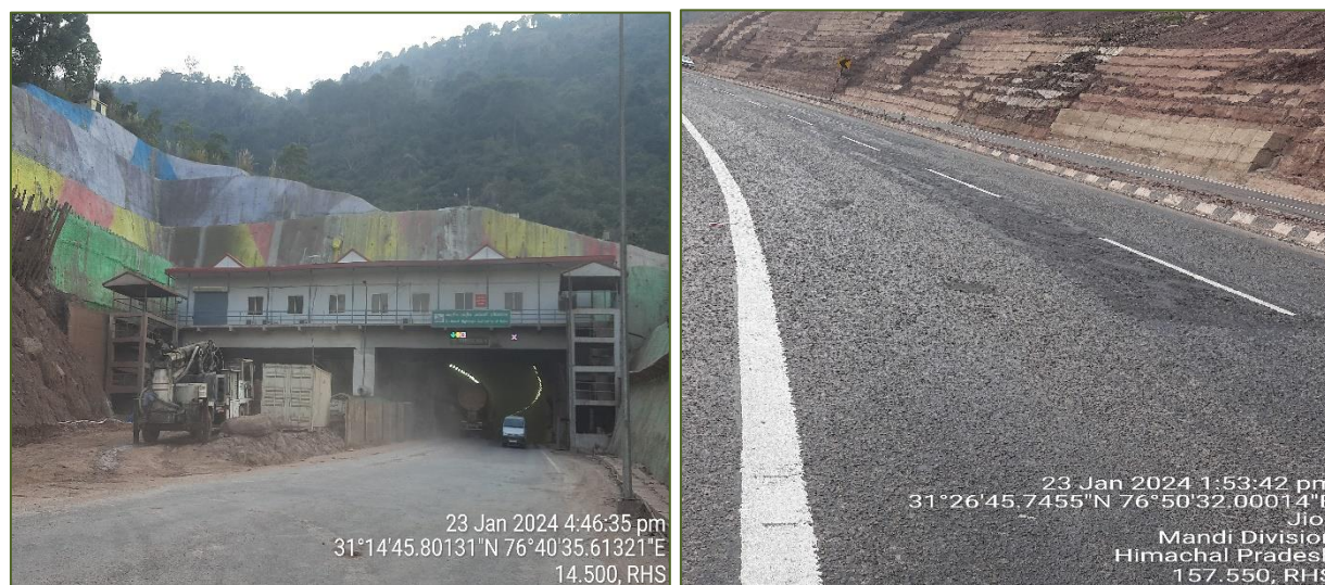
Figure 3-1: Project start and end location
