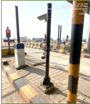
Figure 3-13: LPIC and ICS Cameras.
