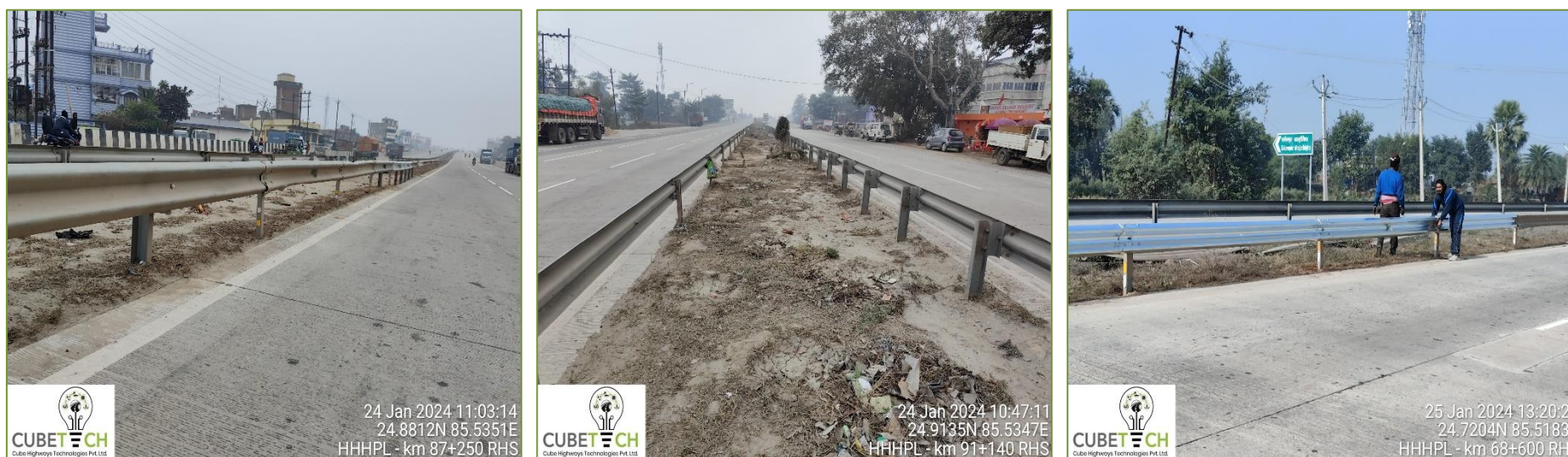
Figure 3-5: Metal beam crash barrier (MBCB) along the project stretch
