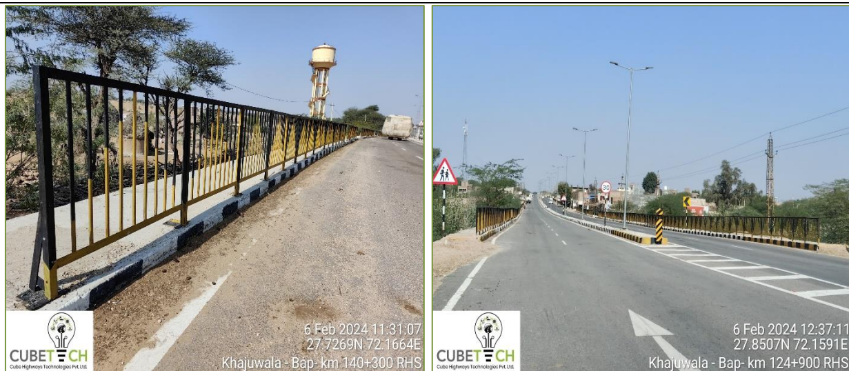
Figure 3-7: Pedestrian guard rail
