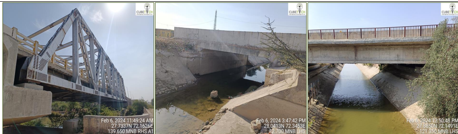
Figure 4-1: Condition of Minor Bridges
