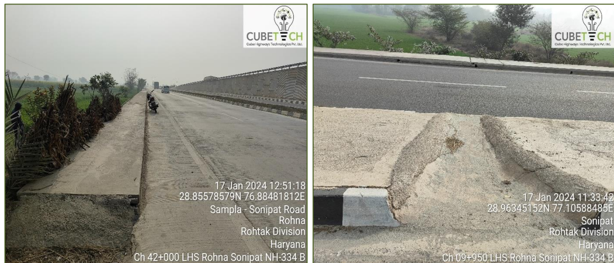
Figure 3-2: Drains
