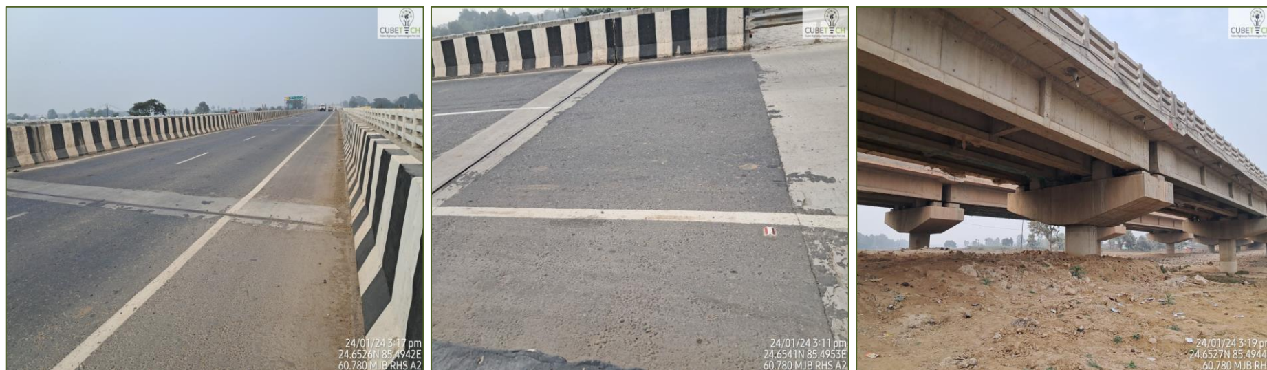
Figure 4-1: Condition of Major Bridges
