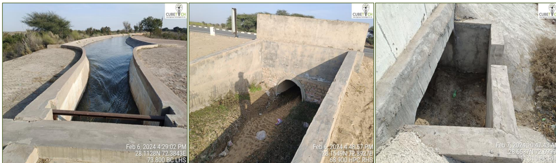
Figure 4-3: Condition of Box Culverts
