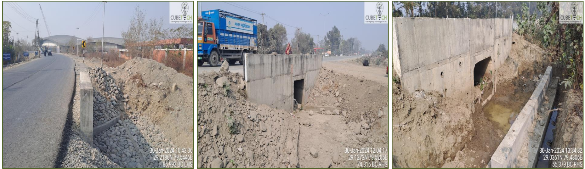
Figure 4-6: Condition of Culverts
