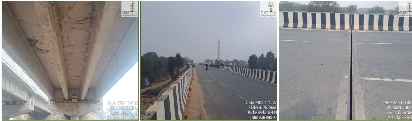
Figure 4-1: Condition of Major Bridges
