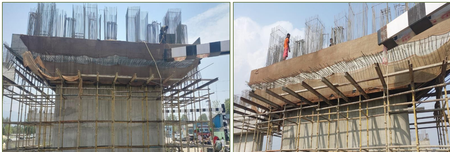
Figure 4-3: Progress of ROB
