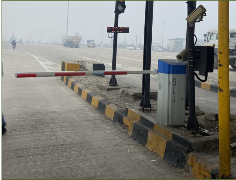
Figure 3-12: Boom Barrier.
