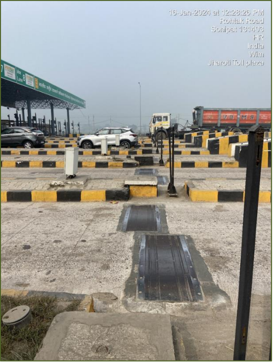
Figure 3-17: Medium Speed Weigh in Motion (MSWIM).
