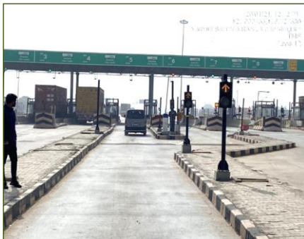
Figure 3-14: Over Head Lane Signal (OHLS).
