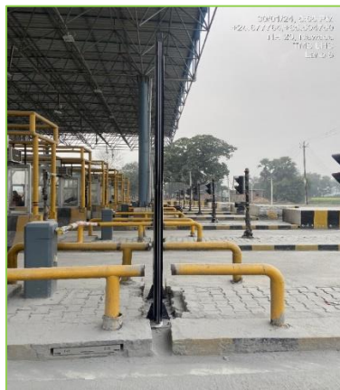
Figure 3-17: AVC Profiler.
