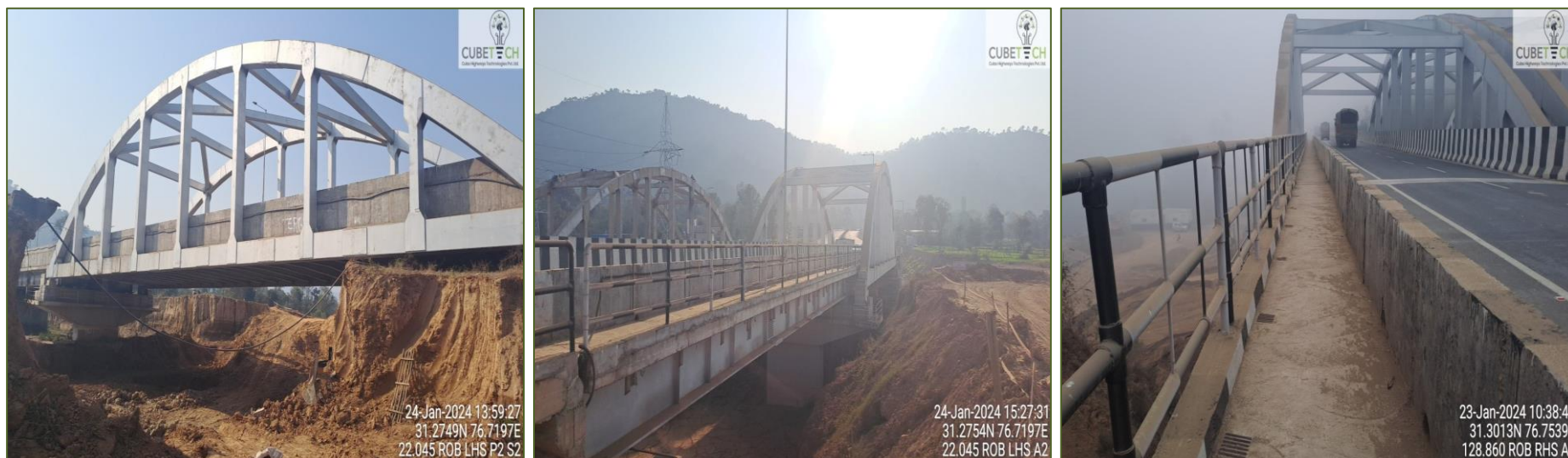
Figure 4-3: Condition of Road Over Bridges
