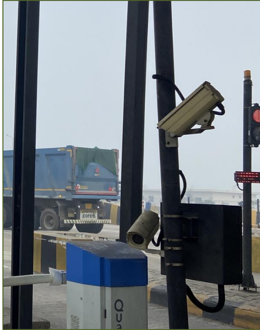
Figure 3-14: LPIC and ICS Cameras.
