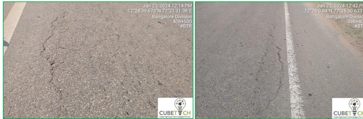
Figure 7-7: Alligator Cracks
