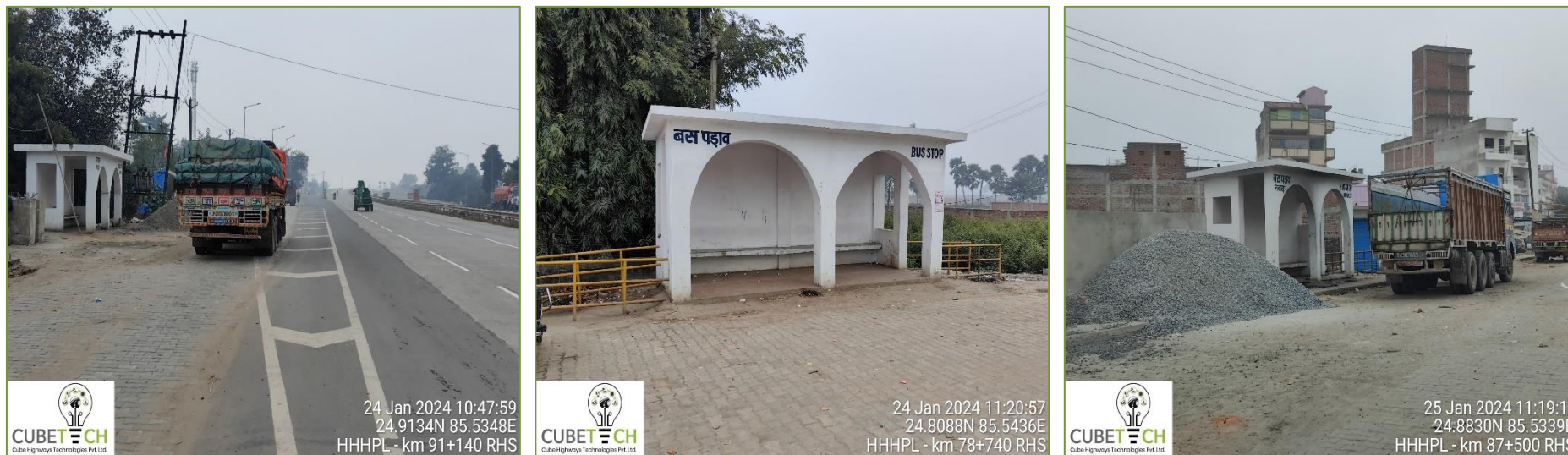
Figure 3-9: Bus bays / shelters
