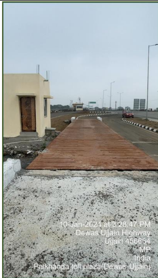
Figure 3-23: Static Weigh Bridge
