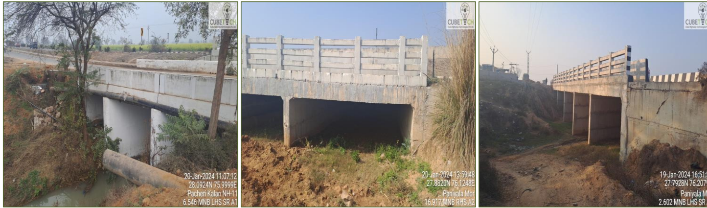
Figure 4-2: Condition of Minor Bridges
