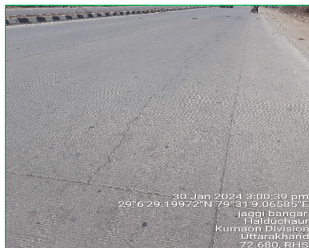
Figure 0-1: Longitudinal Cracks
