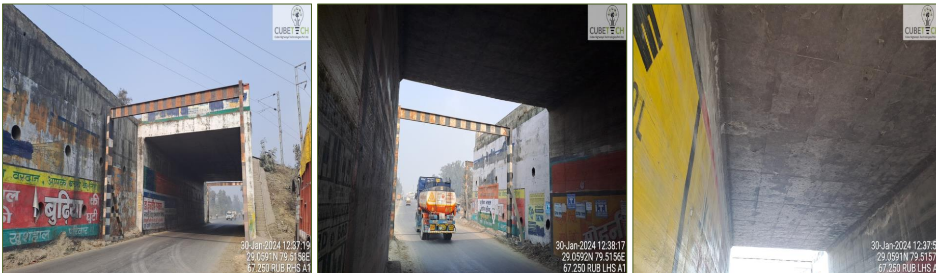
Figure 4-4: Condition of RUB
