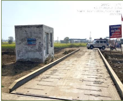
Figure 3-16: Static Weigh Bridge (SWB).
