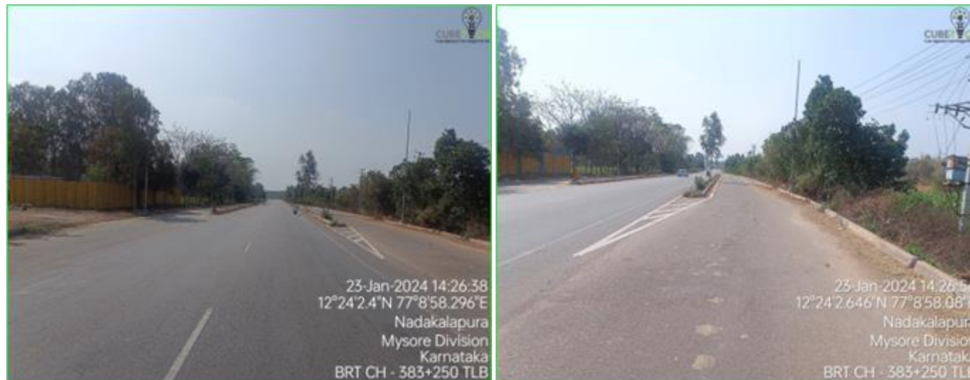
Figure 3-8: Truck Lay bye
