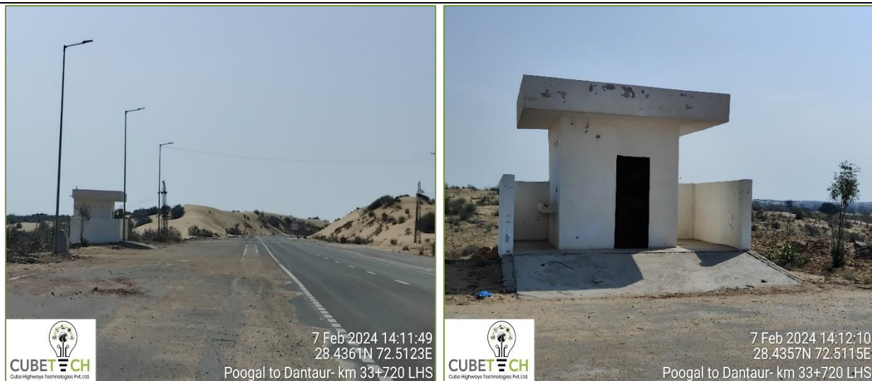
Figure 3-11: Truck Lay bye
