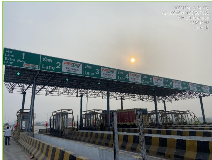
Figure 3-21: Over Head Lane Signal (OHLS).
