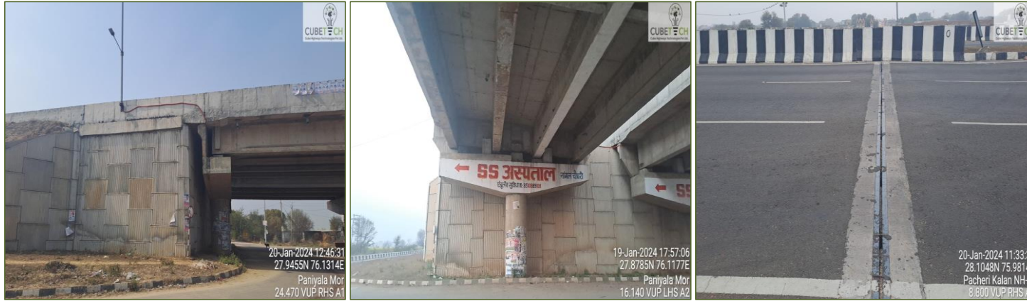
Figure 4-3: Condition of Vehicular Underpasses
