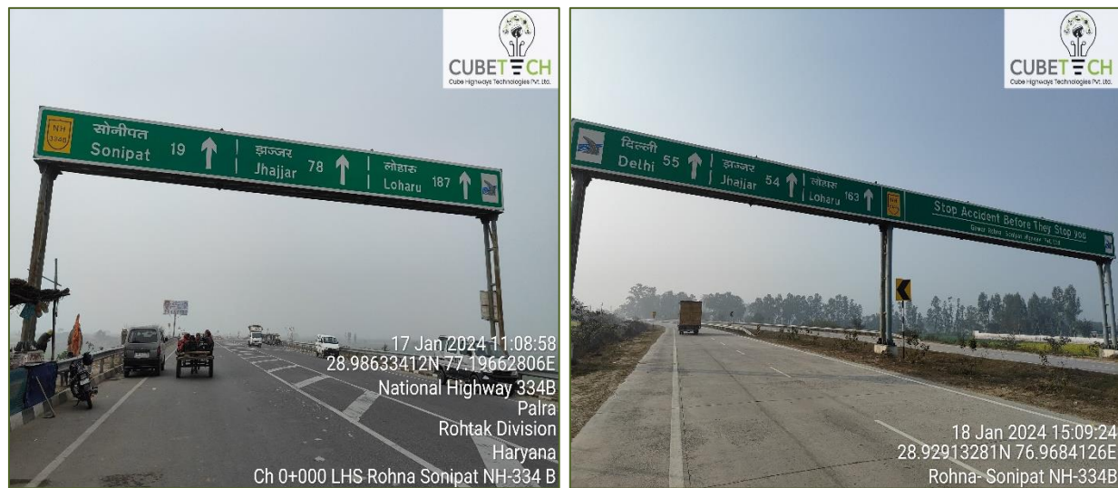
Figure 3-5: Overhead & Cantilever Gantry boards and VMS
