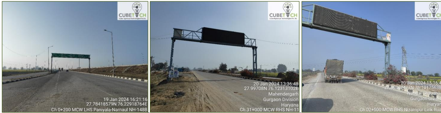
Figure 3-5: Overhead & Cantilever Gantry boards
