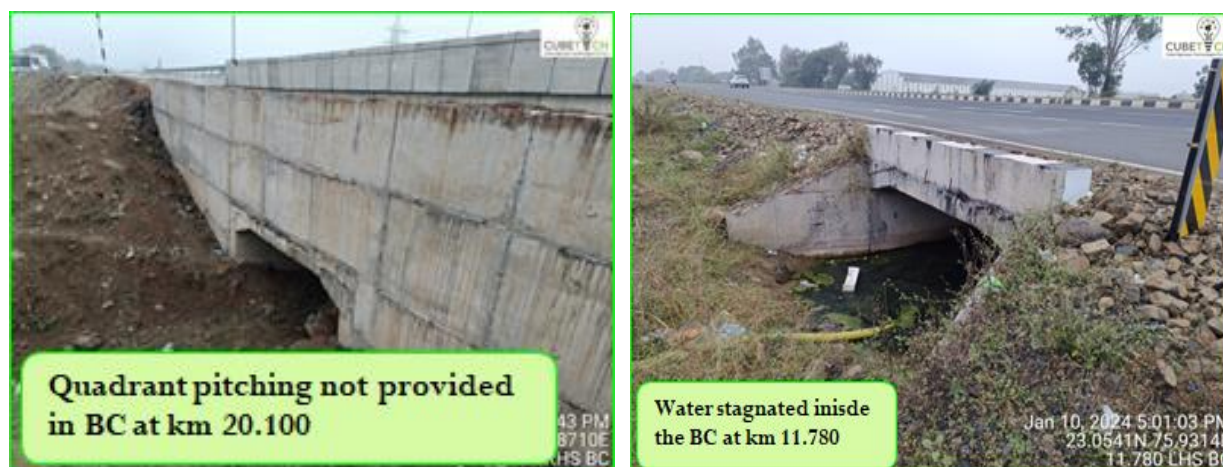
Figure 4-8:.Condition of Culverts
