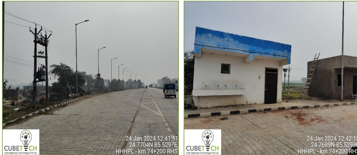
Figure 3-10: Truck Lay bye
