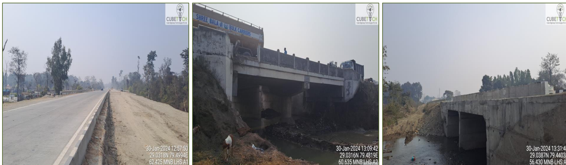
Figure 4-2: Condition of Minor Bridges
