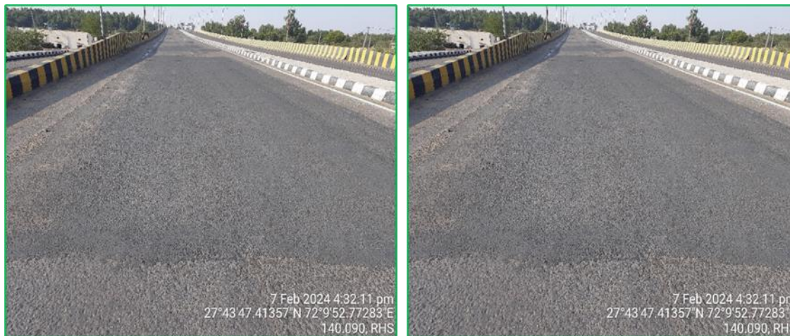
Figure: Patches
