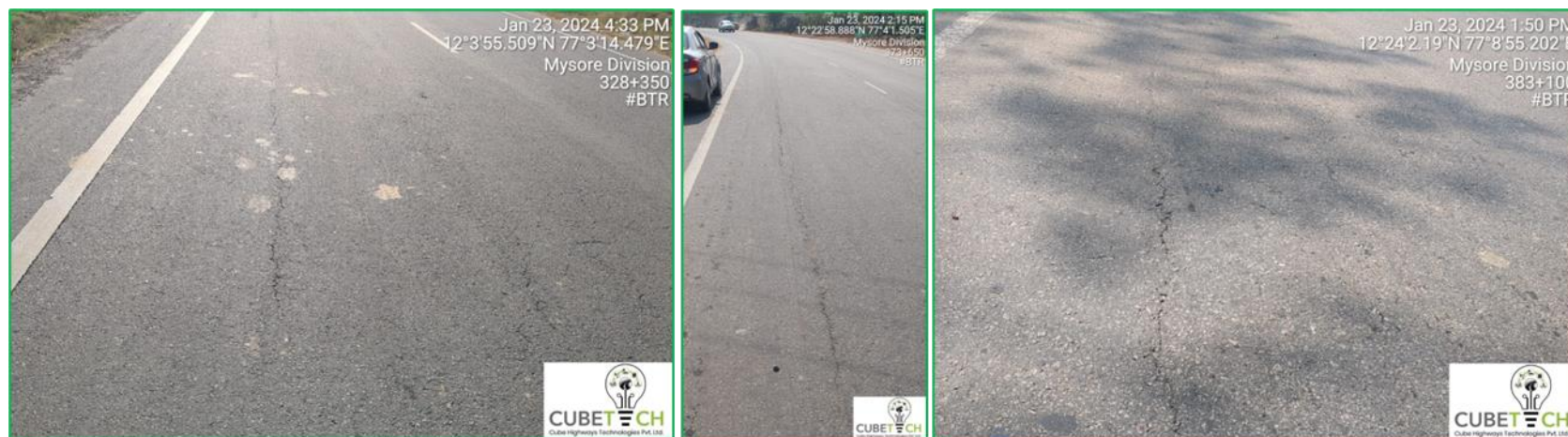
Figure 7-6: Longitudinal Cracks
