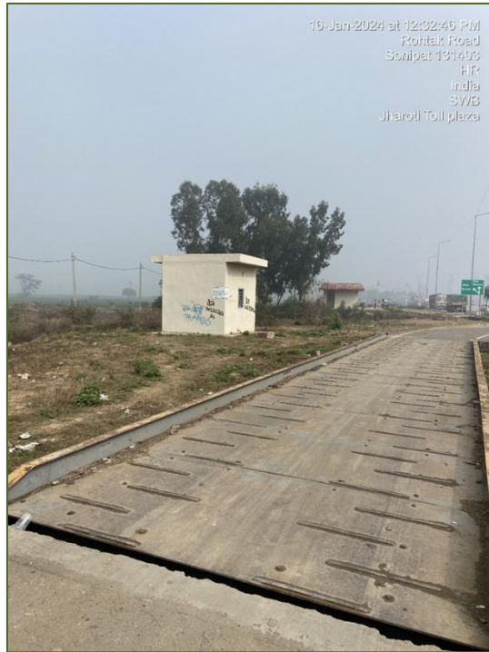
Figure 3-18: Static Weigh Bridge (SWB).
