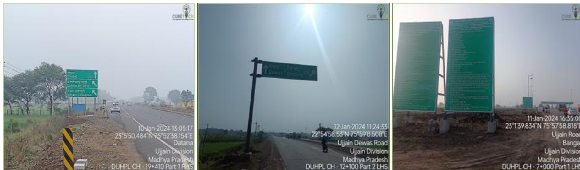
Figure 3-8: Traffic sign boards
