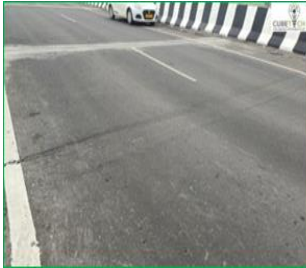
Figure 7-6: Transverse cracks
