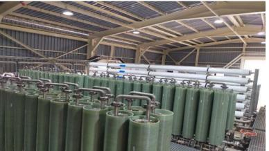
membrane systems help mitigate this by reducing the evaporator load, thereby decreasing steam consumption and lowering operating costs.
