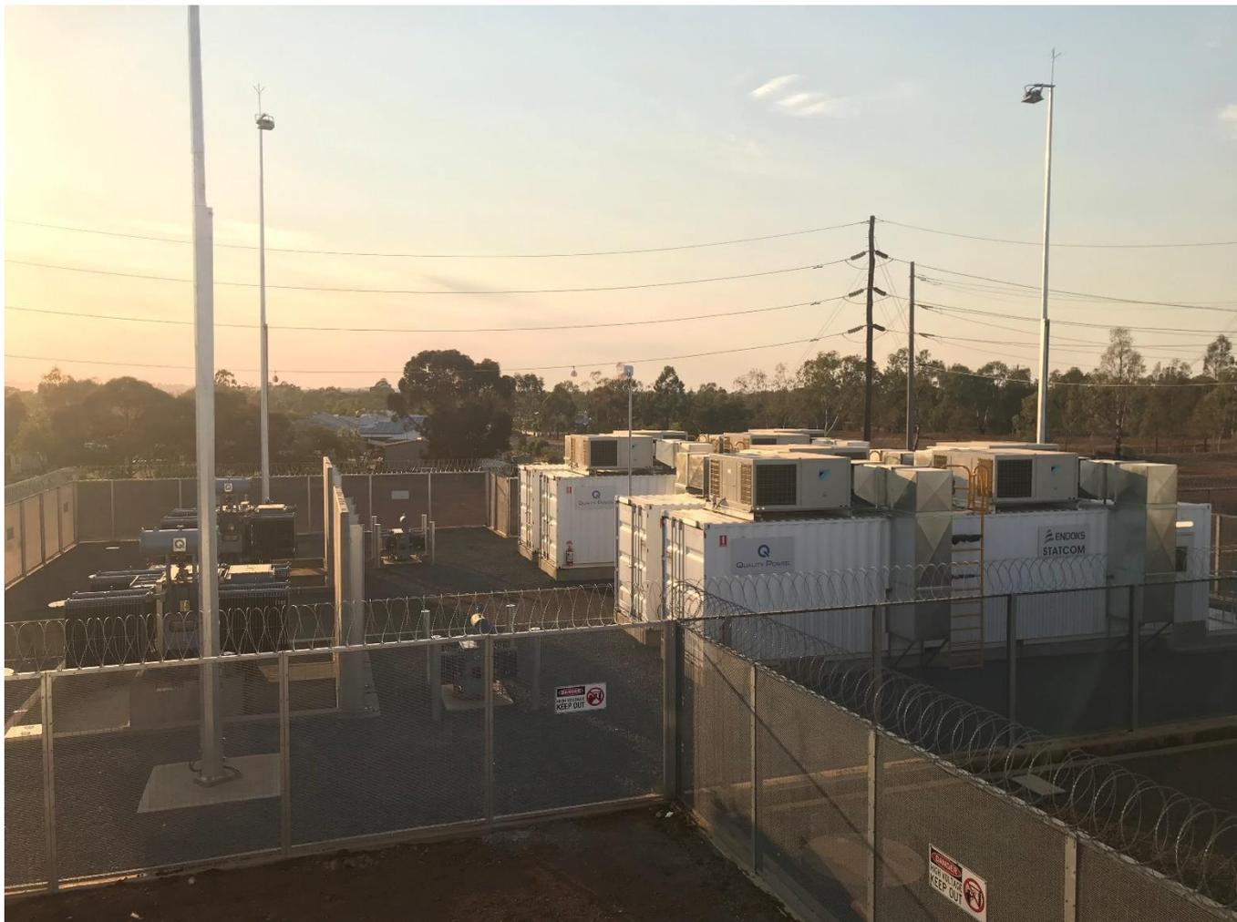
Static synchronous compensator (“STATCOM”) are power electronic devices consisting of voltage-source converters that generate or absorb reactive power as needed to stabilize the voltage of the power system. Unlike traditional SVCs which use thyristor-based technology, STATCOMs utilize insulated-gate bipolar transistors to control the flow of reactive power.
