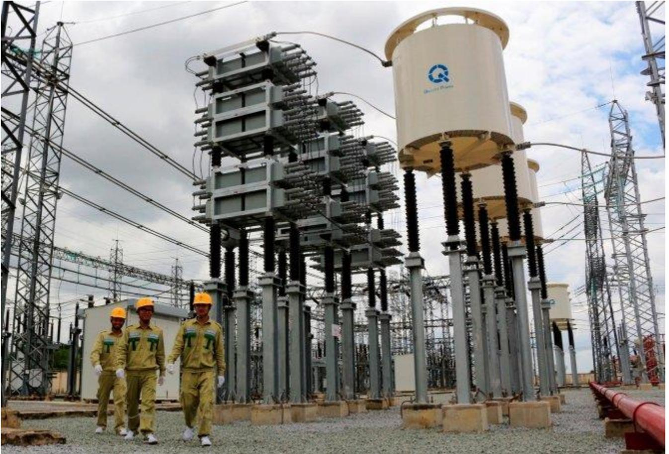
Capacitor banks are electrical devices designed to improve power factor and voltage stability in electrical power systems. They consist of a series of capacitors connected in parallel with the electrical distribution system. Capacitor banks are commonly used in industrial, commercial, and utility settings to compensate for reactive power and enhance overall system efficiency.
