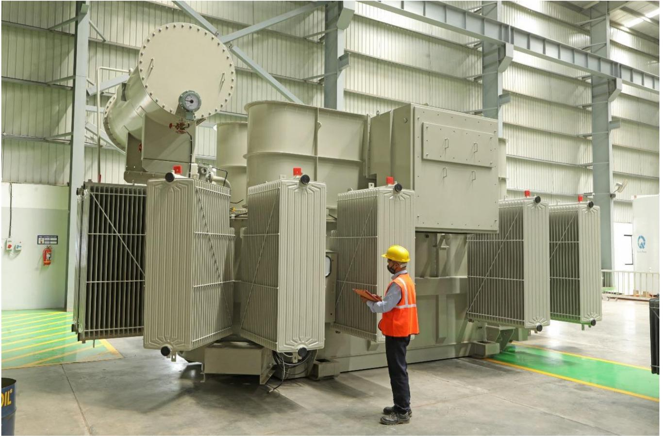
Shunt reactors are vital components used in electrical power systems to stabilize voltage levels and compensate for capacitive reactive power. They are typically connected in parallel with transmission lines or distribution networks and operate continuously to absorb excess capacitive reactive power and thereby maintain voltage within acceptable limits.
