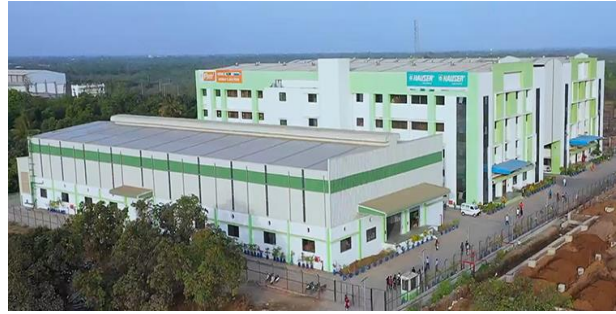
Valsad Building-II and Valsad Building-III
