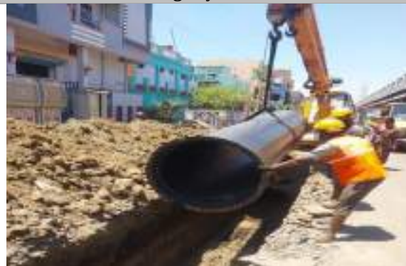
UGSS works at Tondiarpet, Chennai
