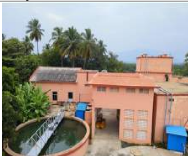
11 MLD & 3.15 MLD Water Treatment Plant at Gobichettipalayam
