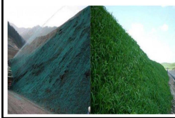
Hydroseeding is the process of mechanically spraying slurry of suitable mixture of seeds, mulch and other ingredients so that barren slopes can be vegetated. Left side is the photo showing the spraying
