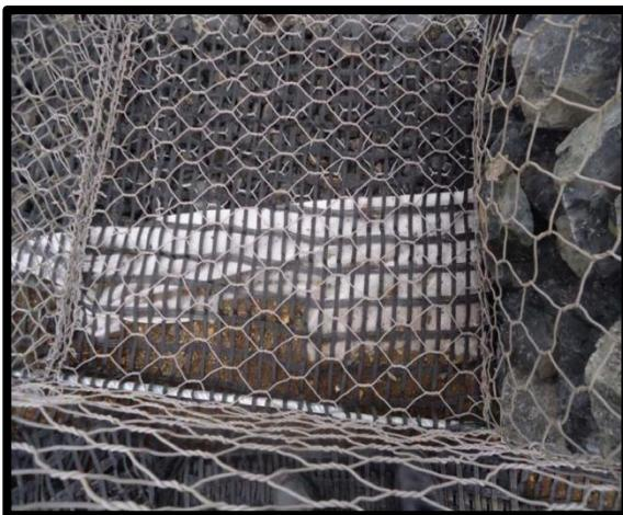
A site photo of the bodkin connection (with cross rod) between gabion and geogrid developed by us in association with IIT Madras. This connection is essential for the stability
