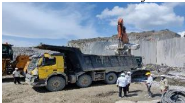
Dump Truck with Excavator in foreground
