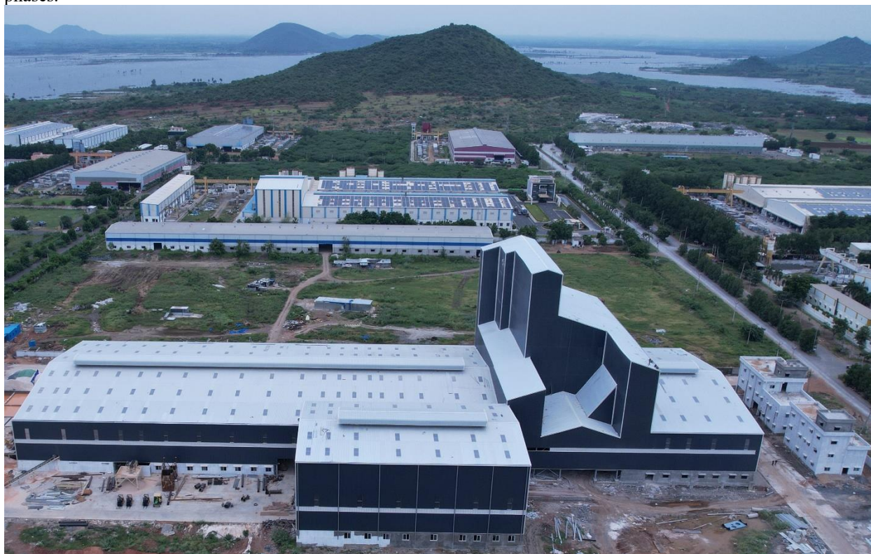
Aerial view of the Phase I Quartz Processing Plant
