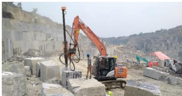
Excavator-mounted Mechanical Drill
