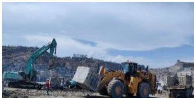
Wheel Loader with Excavator in foreground
