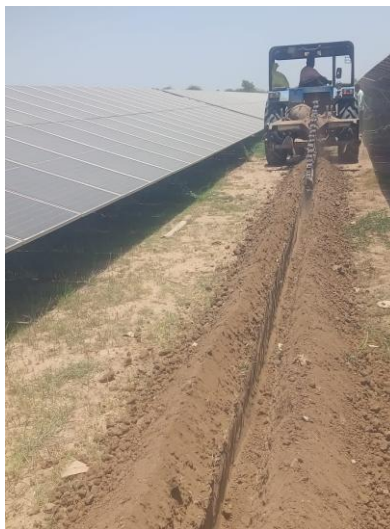
Excavation of Trench
