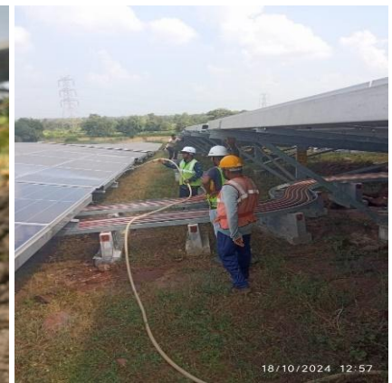
Solar Module Cleaning
