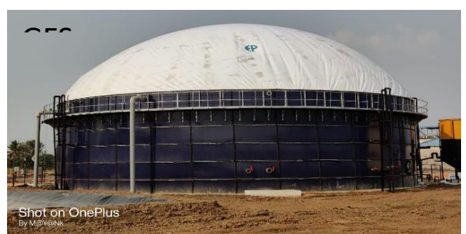
GFS Digester Tank (Completed)
