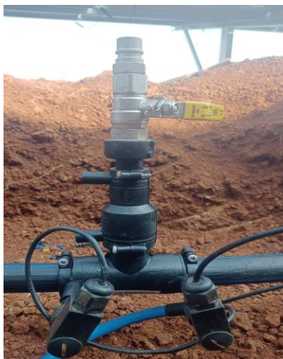
Electrofusion Jointing
