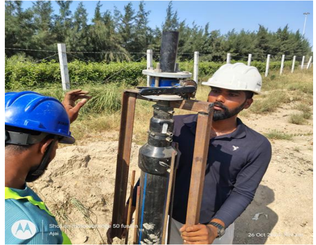
Joining Pipes and Other Related Fittings
