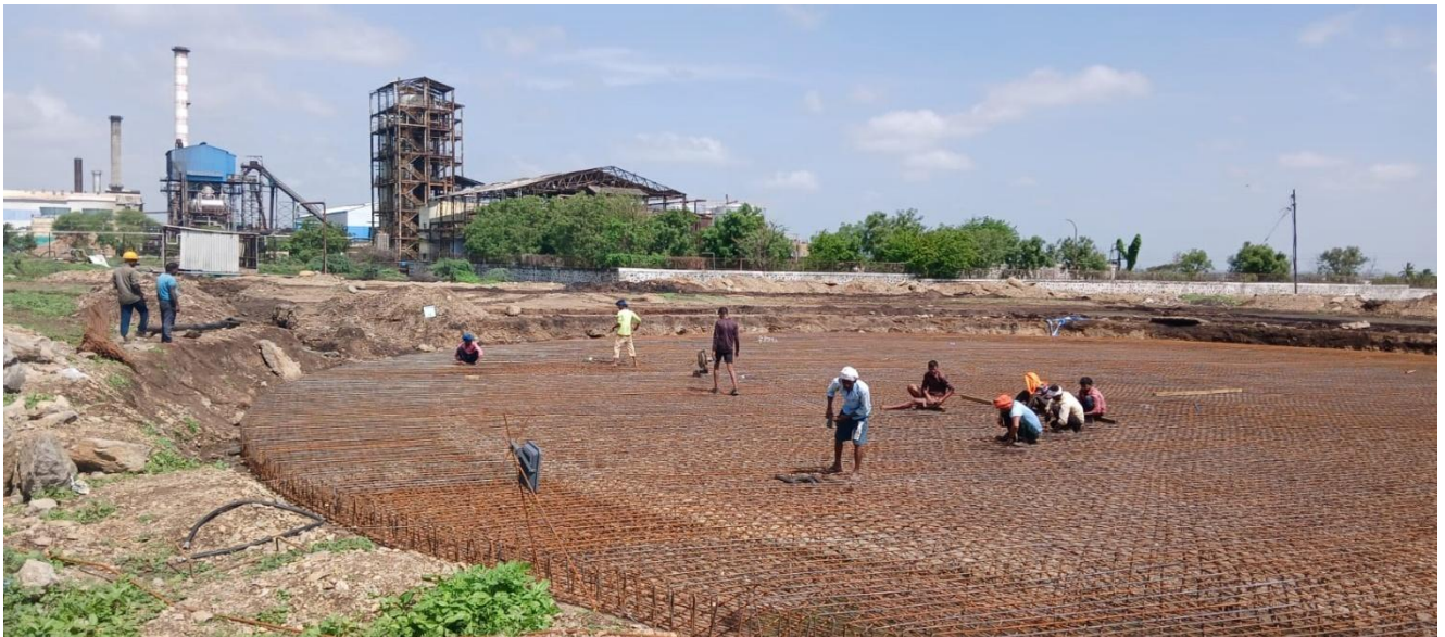
Compressed Bio Gas (CBG) Digester Raft
