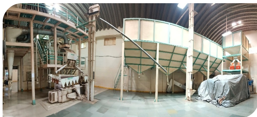
Navrang Cleaning Plant
