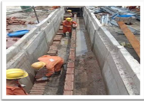
Electric Trench & Brick Work
