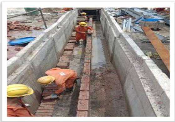
Electric Trench & Brick Work
